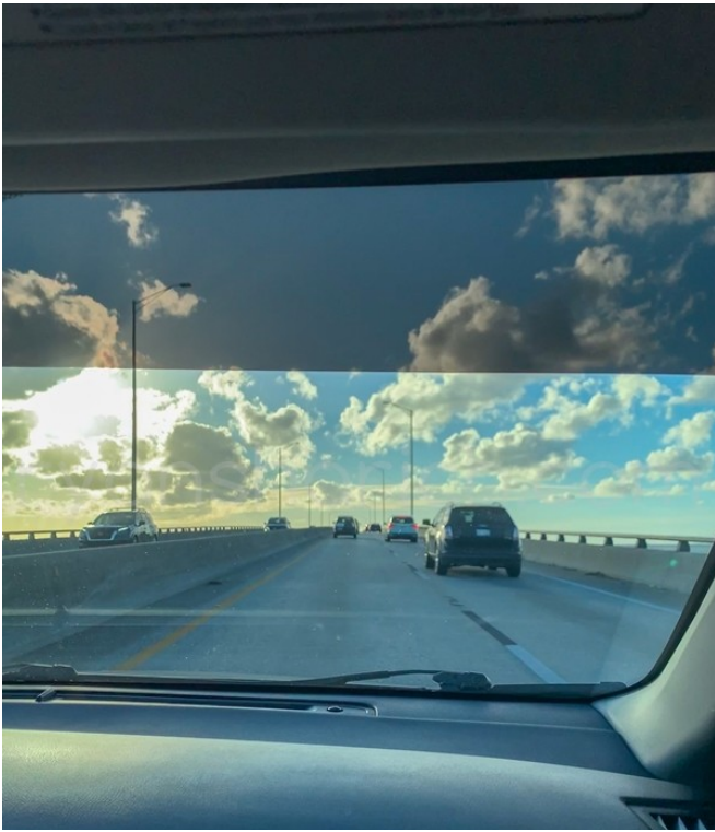
On the Campbell Causeway Road Bridge (State Road 60) over Old Tampa Bay
